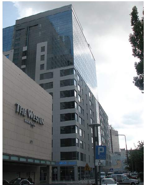
Photo 7. The Atrium City. The view from western side (the photo by the author)
