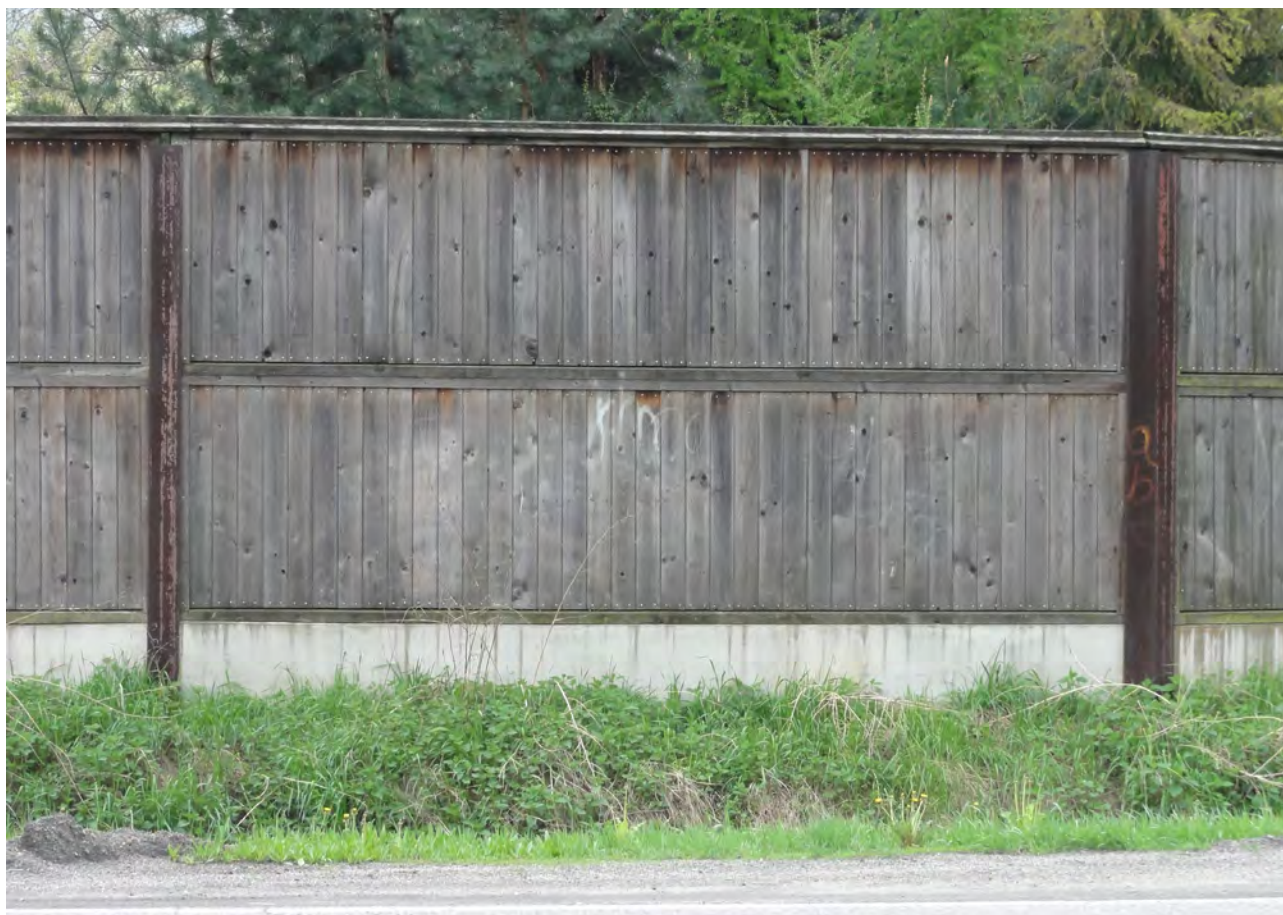
Fig. 1. Timber noise barrier with a board panel (authors' photography)
