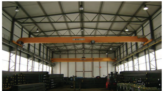
Fig 1. A steel industrial hall with overhead crane handling systems [2]
