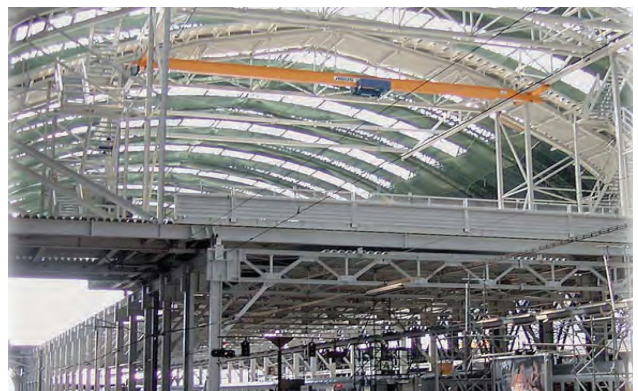
Fig 2. A steel industrial hall with suspended gantry crane handling systems [3]
