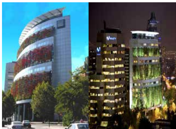
Fig. 2. Consorcio Santiago Building in Santiago de Chile during day and night [14] Rys. 2. Consorcio Santiago Building w Santiago de Chile w dzień oraz w nocy [14]
