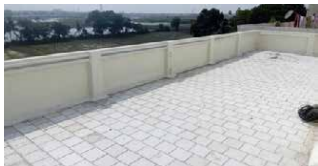
Fig. 4. Roof with mounted cool tiles [17]
