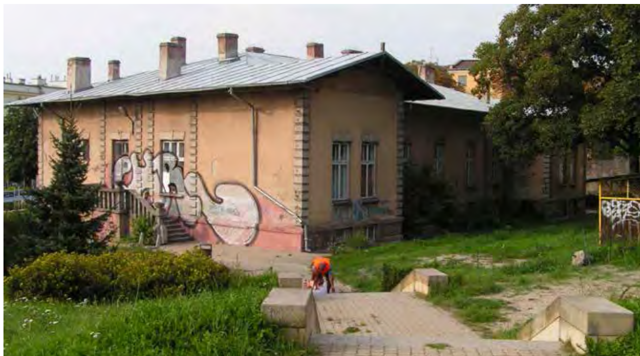
Fig. 13. BWA – Kielce. View from the Castle Hill, the condition of the building before the revitalization. 2011 (Photo by Edyta Banachowska)
