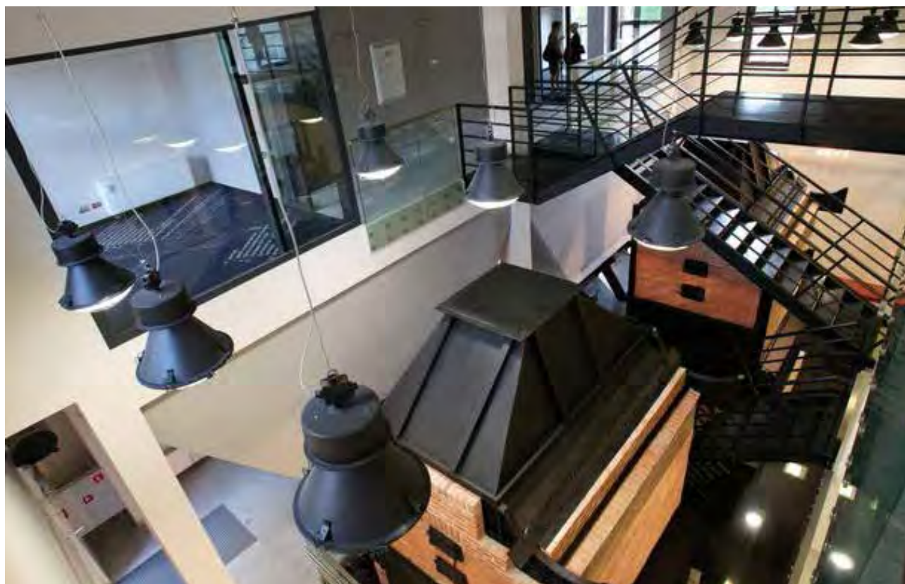
Fig. 10. TEC in Olsztyn. View of the restored La Mont boilers. 2013 (Photo by Tomasz Waszczuk/PAP, source: the Internet)
