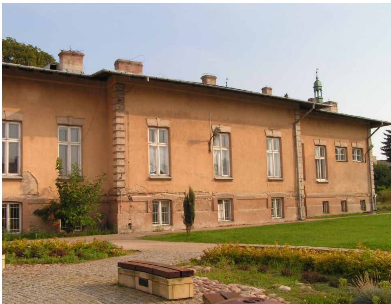
Fig. 12. BWA – Kielce. View from the Artists' Square, the condition of the building before the revitalization. 2011 (Photo by Edyta Banachowska)
