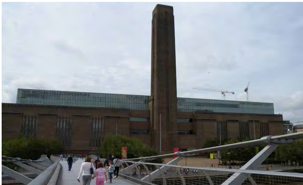
Fig. 1. Tate Modern – London. The condition of the building after the alteration. View from the River Thames and a new footbridge across the river connecting Tate Modern with the northern part of London (Photo by Shaun Jones, source: the Internet)
