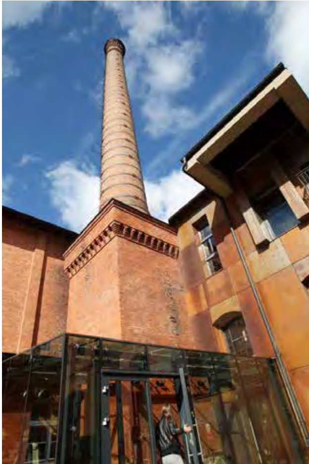
Fig. 11. TEC in Olsztyn. View from the outside, after the alteration. 2013 (Photo by Tomasz Waszczuk/PAP, source: the Internet)
