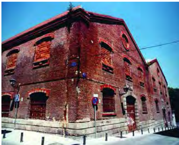
Fig. 4. CaixaForum – Madrid. Power plant building before the restoration works (Photo by Herzog & de Meuron, source: the Internet)
