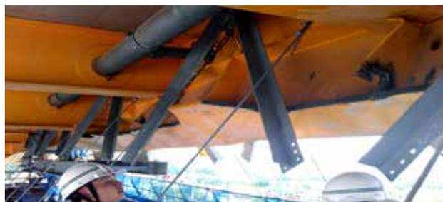
Fig. 4. Main girder deformation after the ship collision with Binh Bridge during CONSON hurricane
