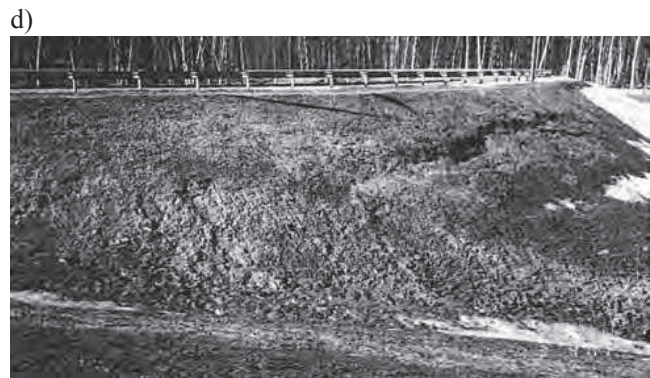
Fig. 1. Local deformations of subgrade embankment: a) road in Alaska [4]; b) Qinghai - Tibet railroads [3]; c) Russia – road «Yamal» [1]; d) Russia – road «Don» 104 km [1]
