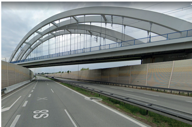
Fig. 1. Side view of the bridge ( https://www.google.com/maps )
