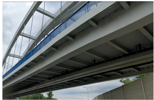
Fig. 2. Bottom view of the bridge ( https://www.google.com/maps )
