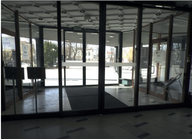
Fig. 5. Main entrance area with glazing markings
