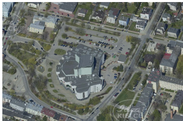
Fig. 2. View of the KCC building
