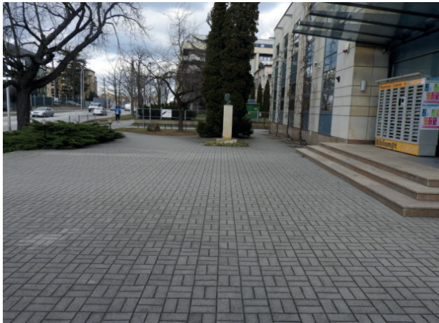
Fig. 11. Pavement zone on the front side
