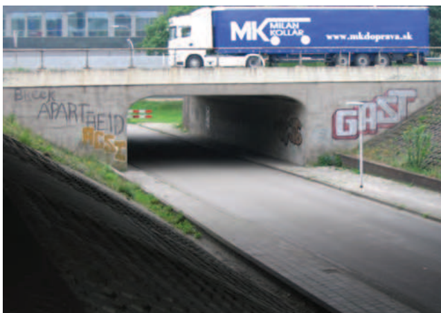
Fig. 3. Solid slab bridge deck
