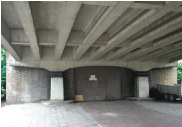
Fig. 2. T-beam bridge deck
